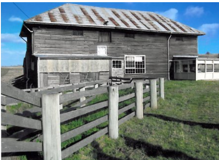
"Wanstead Park" Shearing Shed, Campbell Town, Tasmania
