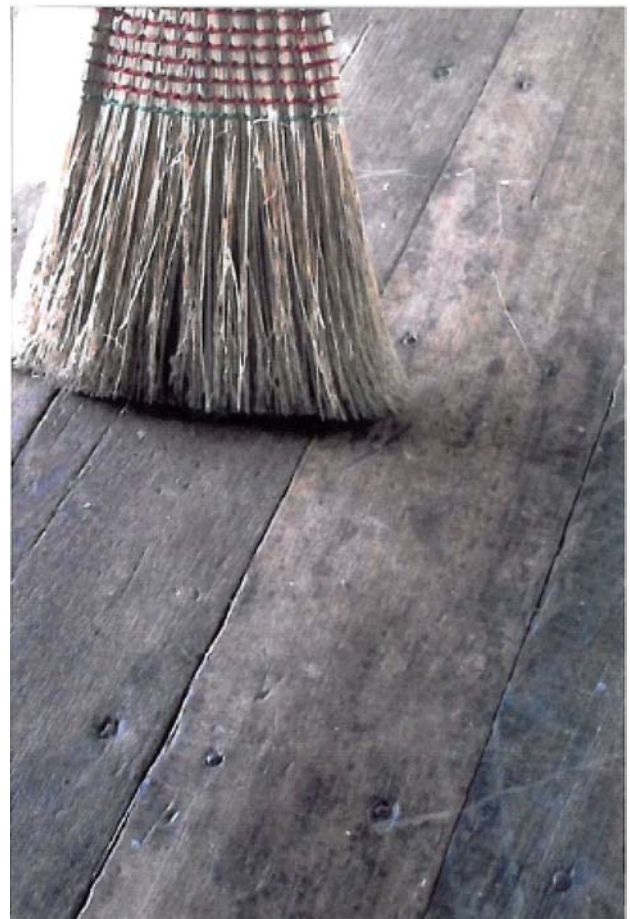
"Wanstead Park" Shearing Shed, width of floor boards.
